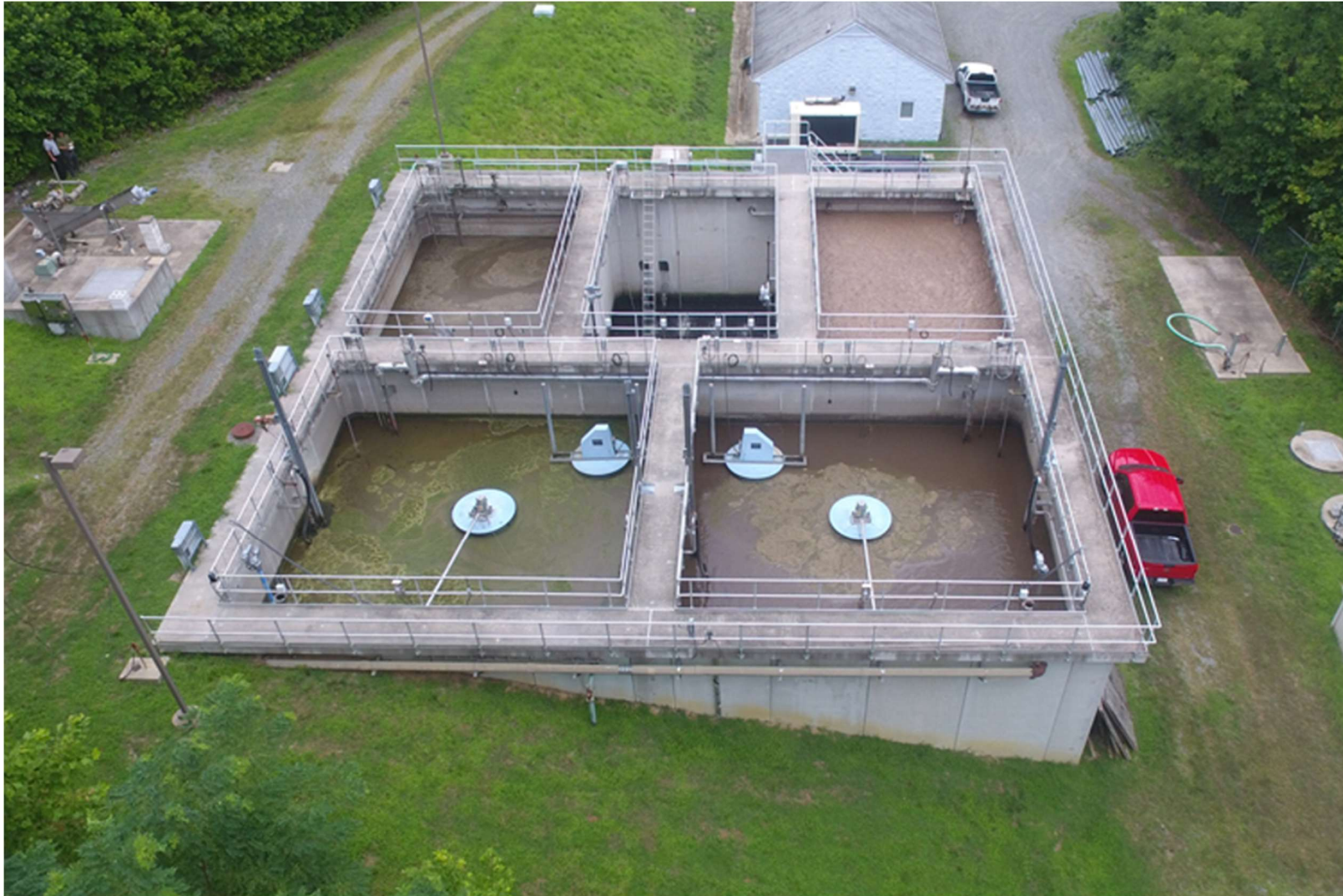
Figure 5. Image of a generic SBR as photographed from above.
